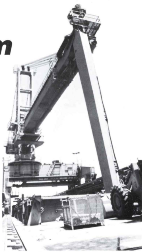
Siwertell unloaders at the Yanbu terminal.
