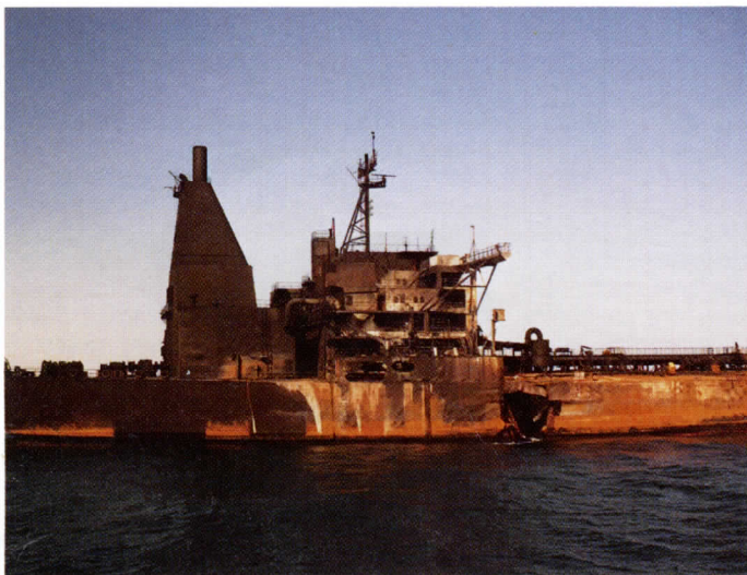
The hole in the starboard side of Safina Al Arab is 20 m 2 .
