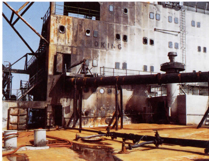
The deck house is completely gutted. The Safina Al Arab is a total loss.
