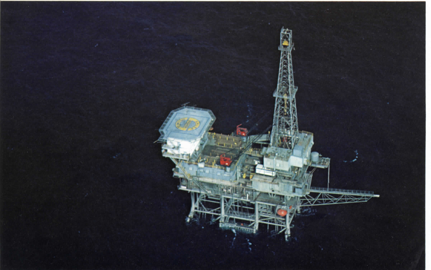
Salenergy III drilling production wells from a platform belonging to TRANSOCO.
